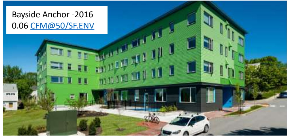
Maine Building Code Blower Door Requirement 0.30 CFM@50/SF.ENV
