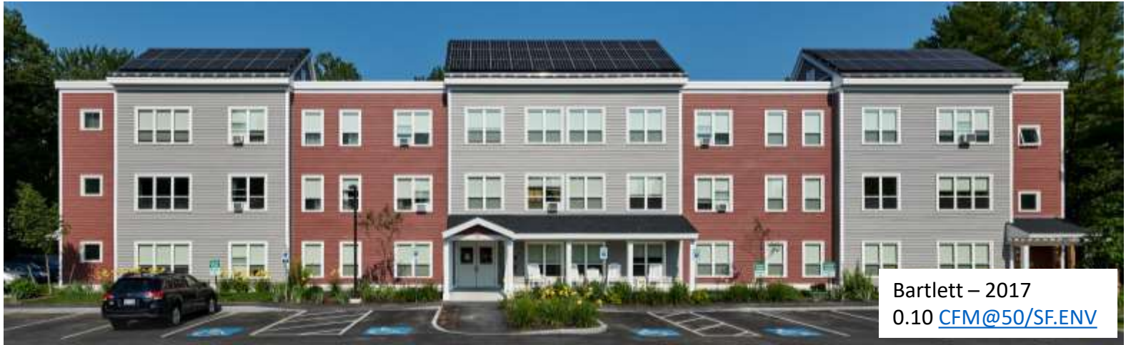
Maine Building Code Blower Door Requirement 0.30 CFM@50/SF.ENV
